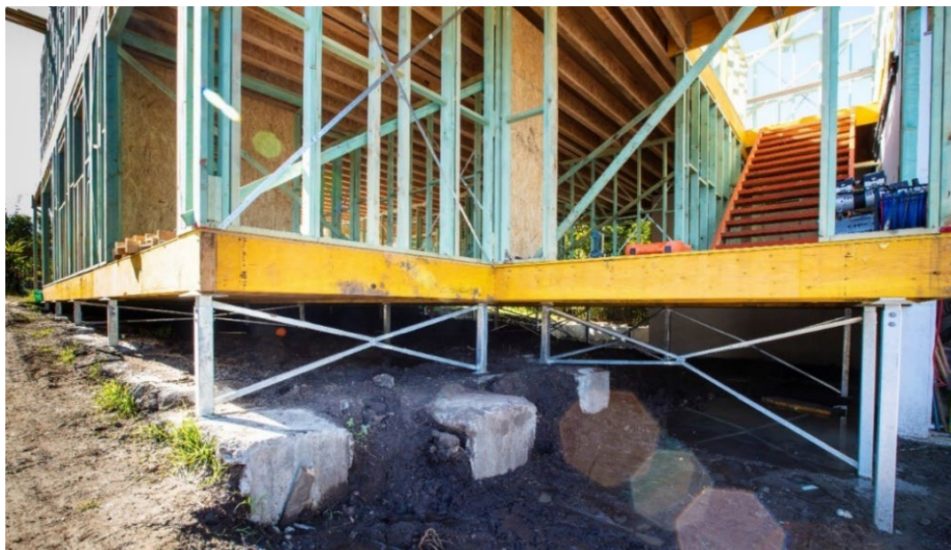
Figure 12 Batch HDG coated posts being used in combination with a traditional timber frame and subfloor.
