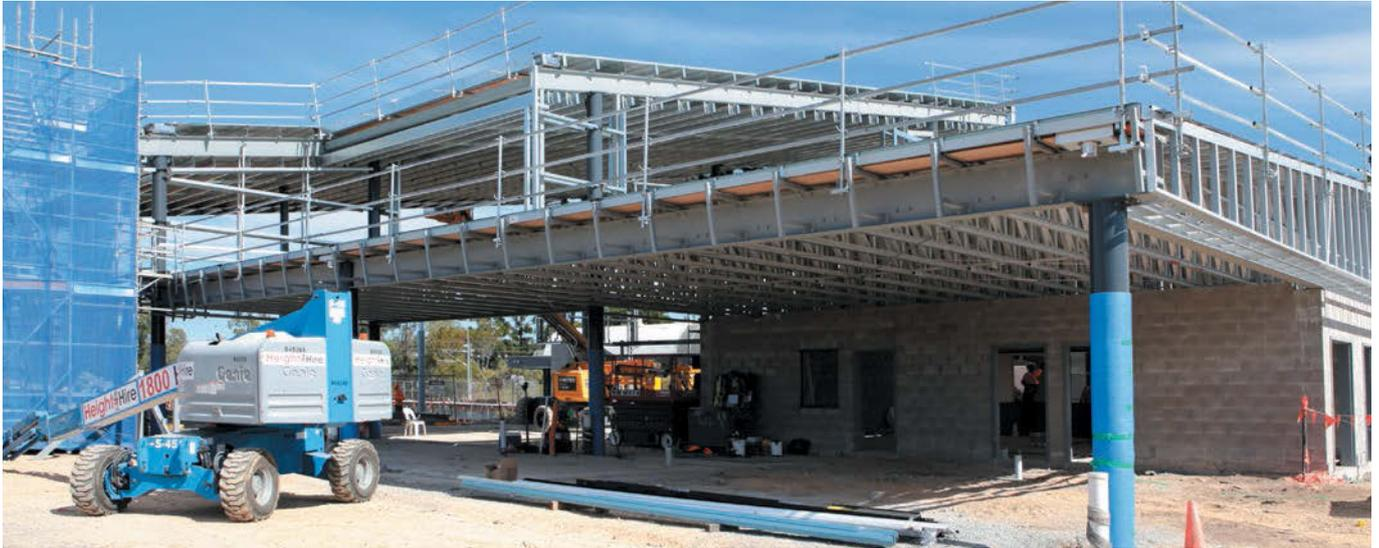
“For the braced bays, piles are required to resist the uplift due to the overturning induced by the lateral load on the building. The uplift values are too large to be resisted by reasonably sized pad footings.”
