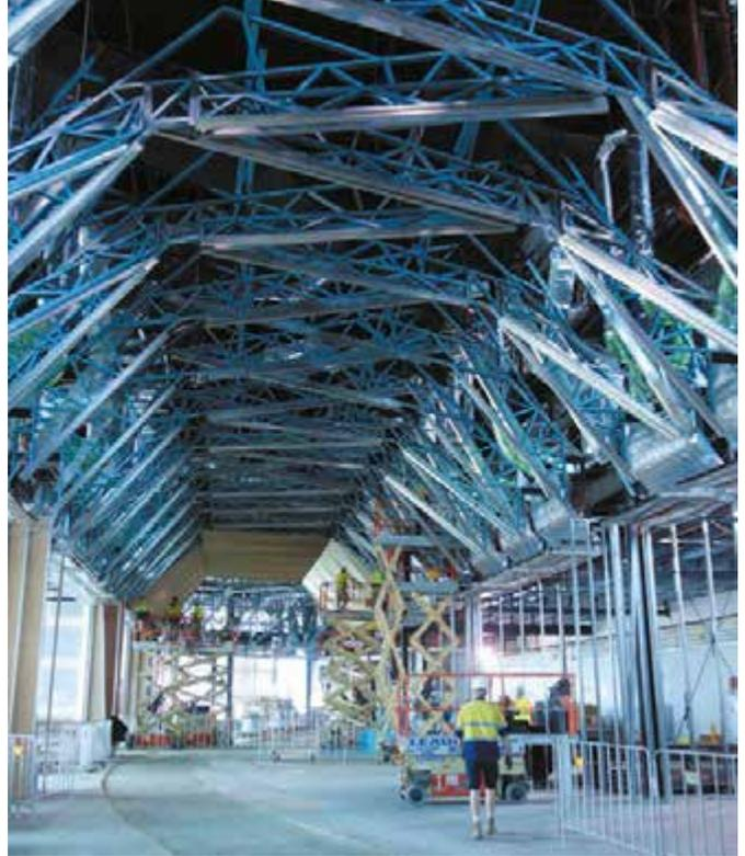
The fabrication was programmed to meet JIT provisions for erection of the steelwork limited to four areas on the busy operating site; the satellite plant platform, high level catwalks, luxury retail framing and walkways, and laneway steelwork.
