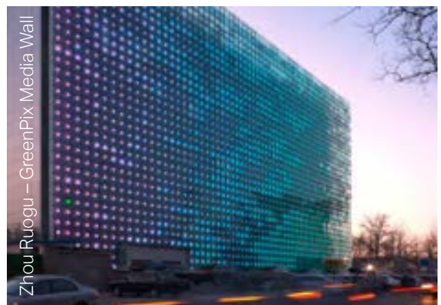
Figure 80: Example of building-integrated photovoltaics
