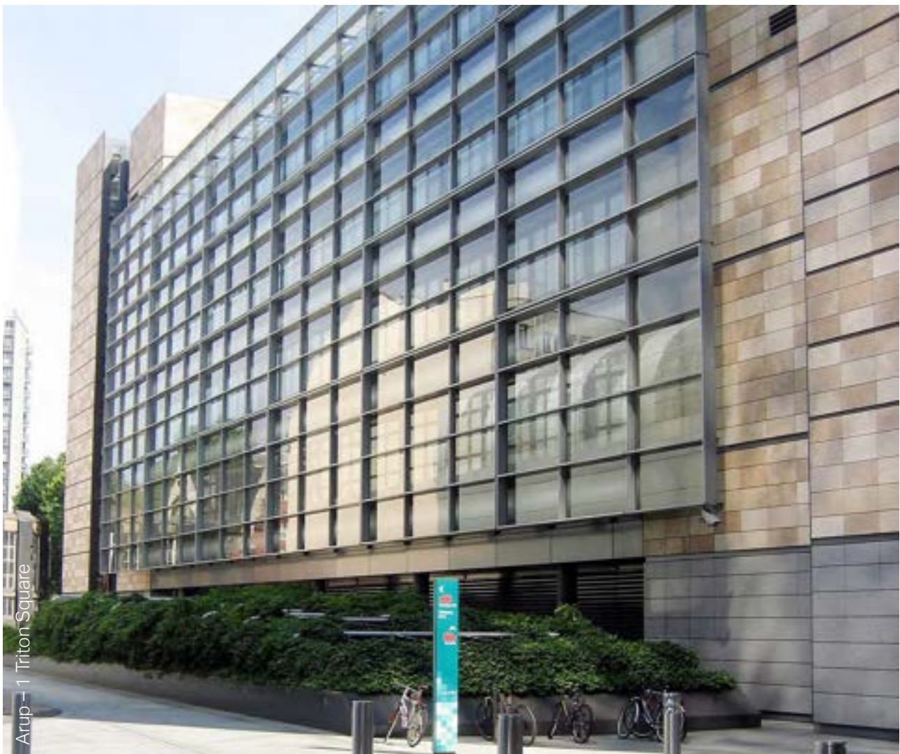
Figure 70: Triton Square, London – 3,000m 2 of façade taken down and refurbished locally to improved performance criteria
