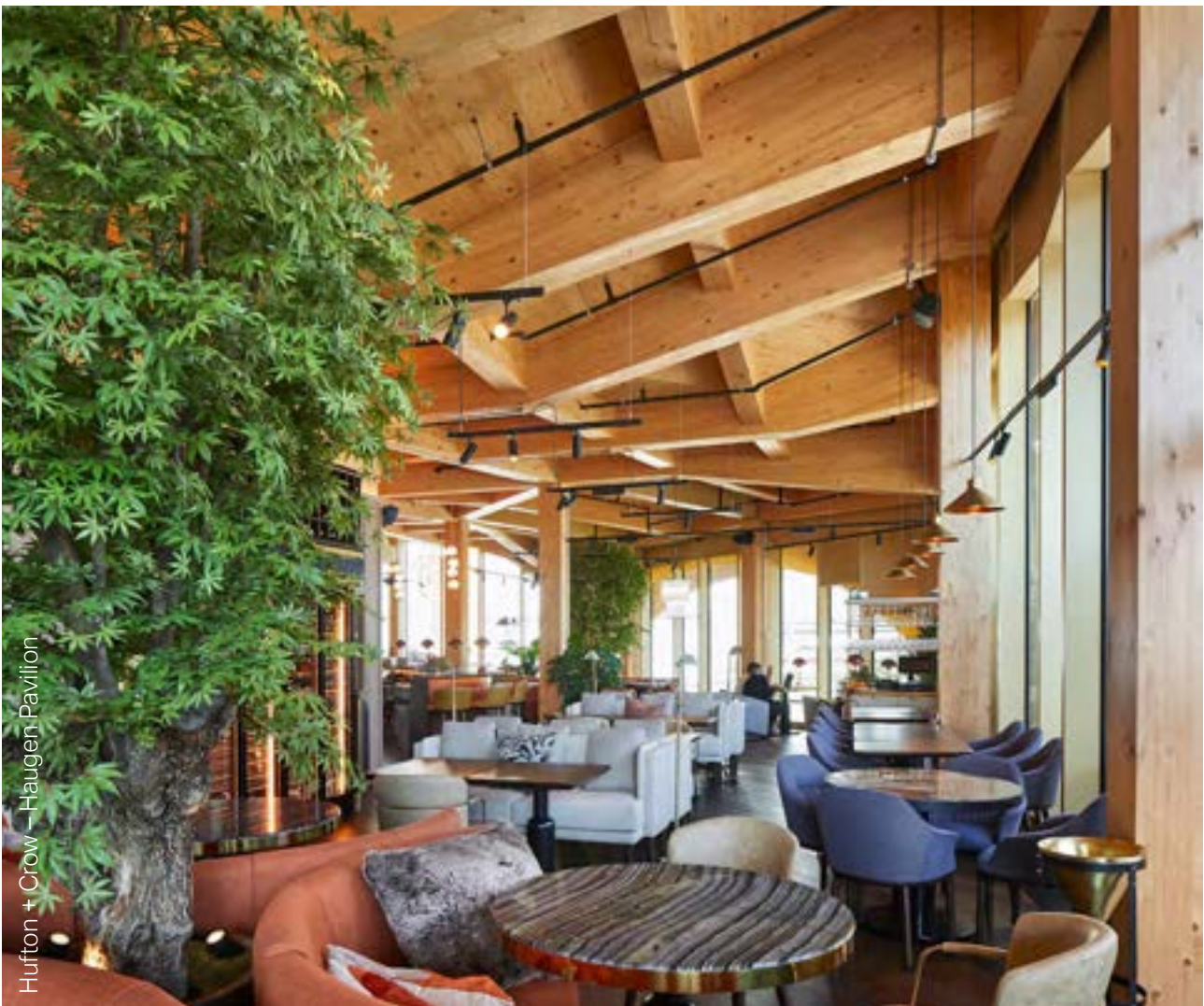
Figure 49: Haugen Pavilion in Stratford, London demonstrating mass timber construction
