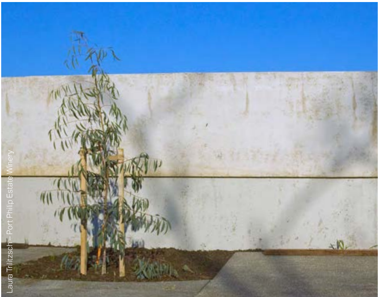
Figure 55: Example of rammed earth wall
