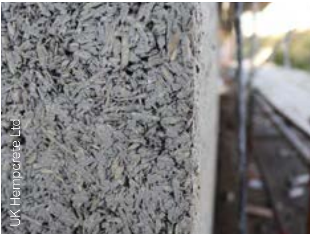
Figure 87: Example of hempcrete wall
