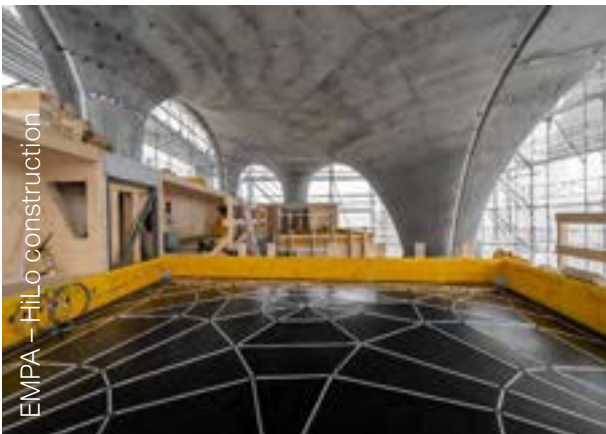
Figure 57: EMPA-ETH Zurich HiLo vaulted flooring system
