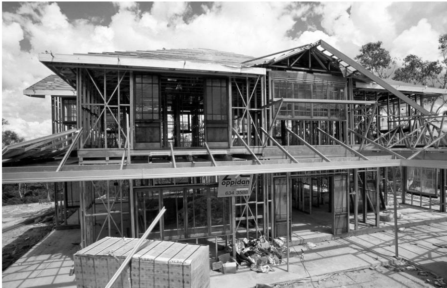
Fig. 1.11 Two-storey steel framed house
