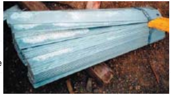
The 'white rust' on these galvanized flat bar sections has been caused by their being wet in the bundle. Galvanized coatings require good ventilation when newly applied to allow the passive oxide films to develop.
