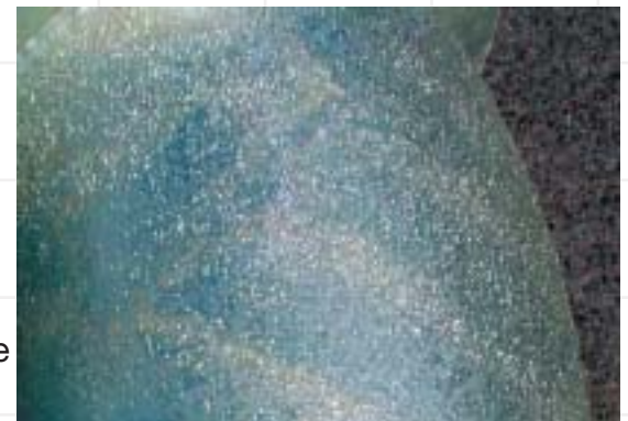
Dross pimples on this pipe spool arise from dross crystals being stirred up from the bottom of the galvanizing bath by long or deep items. Appearance is unsightly but durability is unaffected.
