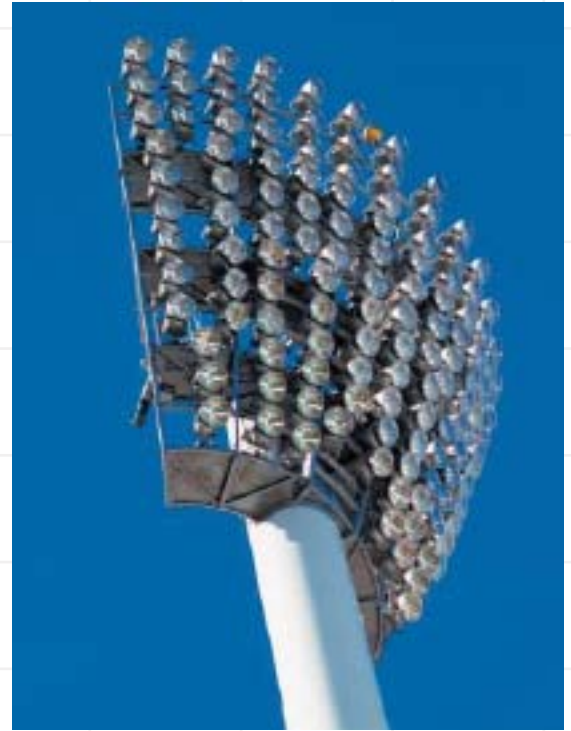
Galvanized stadium lighting poles are usually painted for aesthetics. Properly applied finished add substantially the maintenance free life of the structure.
