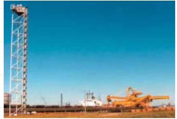
This navigation tower on Newcastle (NSW) Harbour was galvanized and painted to provide additional durability in a marine environment, and remains in good condition after 20 years in service
